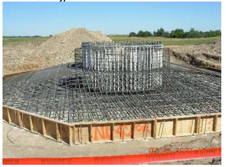
Exhibit 2.6.1 – Typical Turbine Foundation
