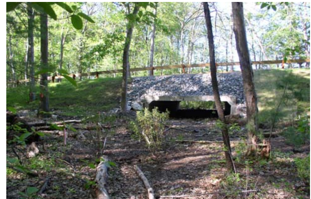
Exhibit 3.2.1 - Bottomless Culvert
