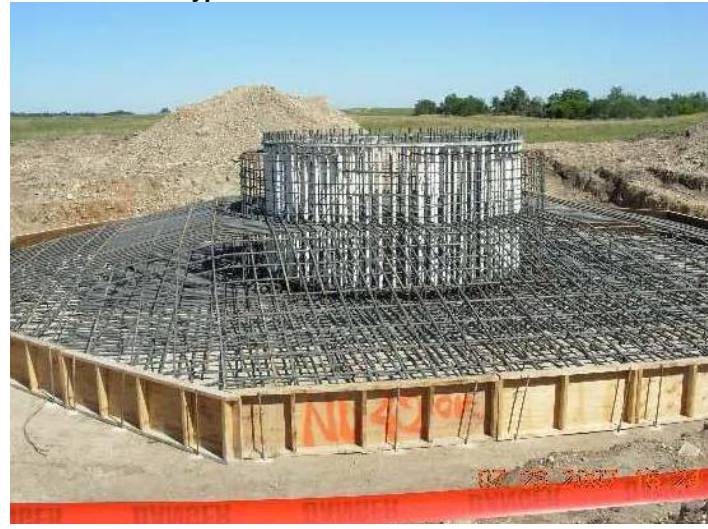
Exhibit 2.6.1 – Typical Turbine Foundation
